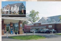
G Gas Station - 2nd Floor Office - Fuel Pumps in Back
