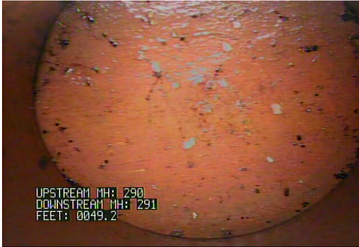
TFC - Tap, Factory Made: Capped @ 49.2 ft.
