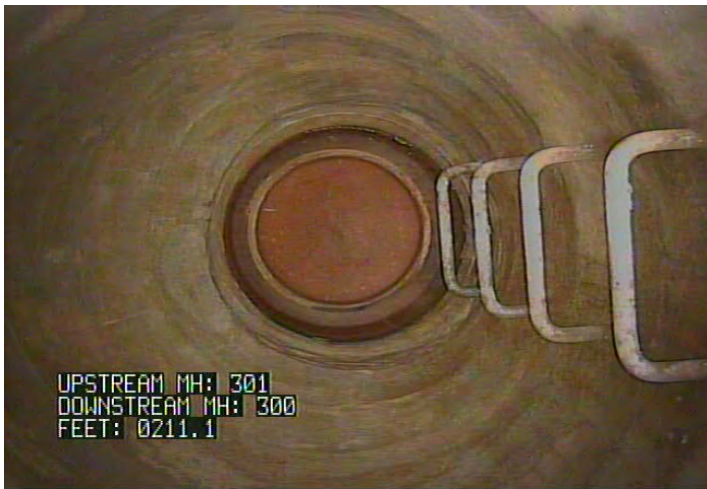
AMH - Access Point - Manhole @ 211.1 ft. MH 300
