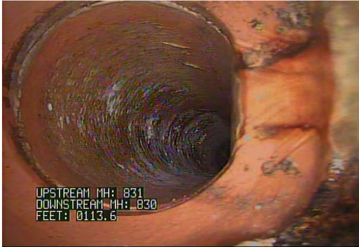
TFA - Tap, Factory Made: Active @ 113.6 ft. DYE PRESENT
