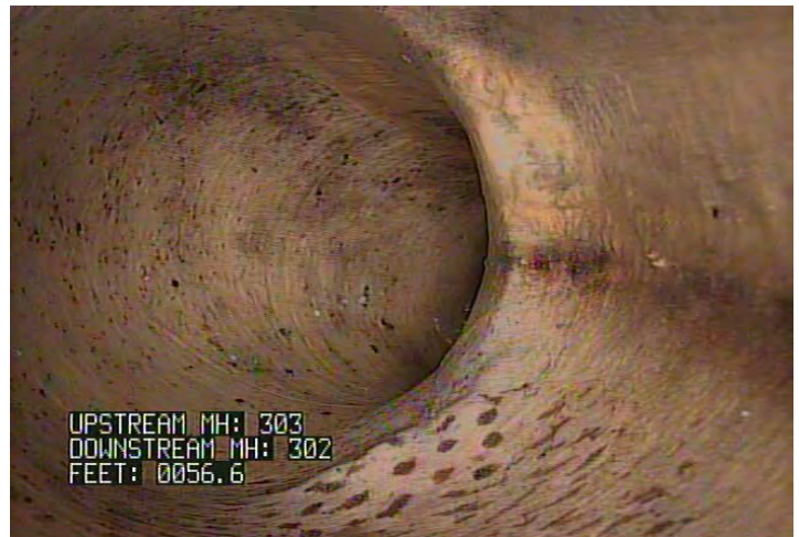
TF - Tap, Factory Made @ 56.6 ft. (CIPP) T LINER
