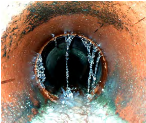
Figure 1.2 Example of Infiltration
