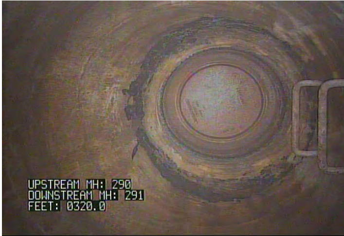
AMH - Access Point - Manhole @ 320.0 ft. MH 291
