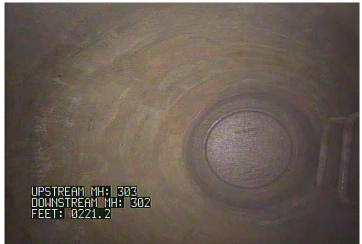
AMH - Access Point - Manhole @ 221.2 ft. MH 302
