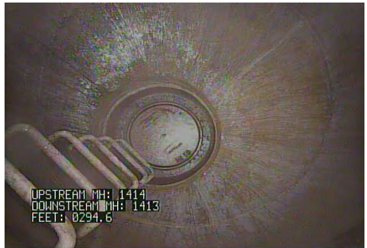
AMH - Access Point - Manhole @ 294.6 ft. MH 1413
