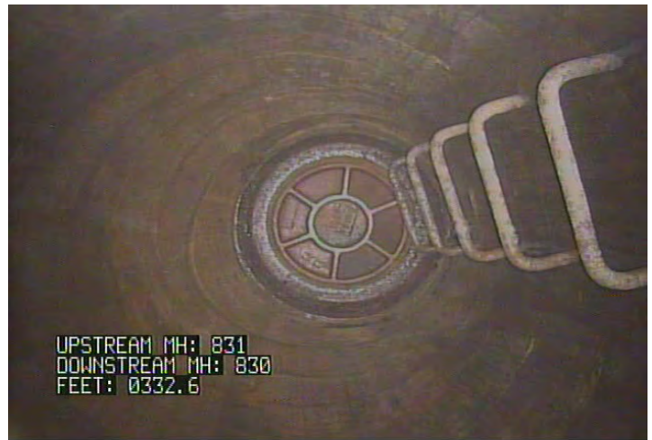
AMH - Access Point - Manhole @ 332.6 ft. MH 830
