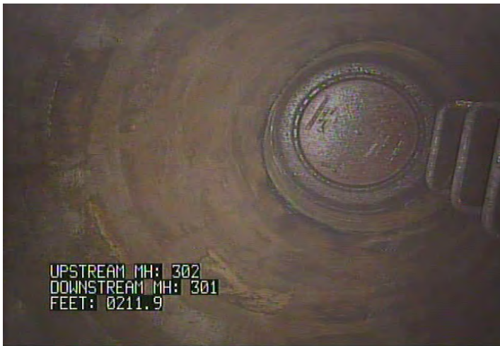
AMH - Access Point - Manhole @ 211.9 ft. MH 301
