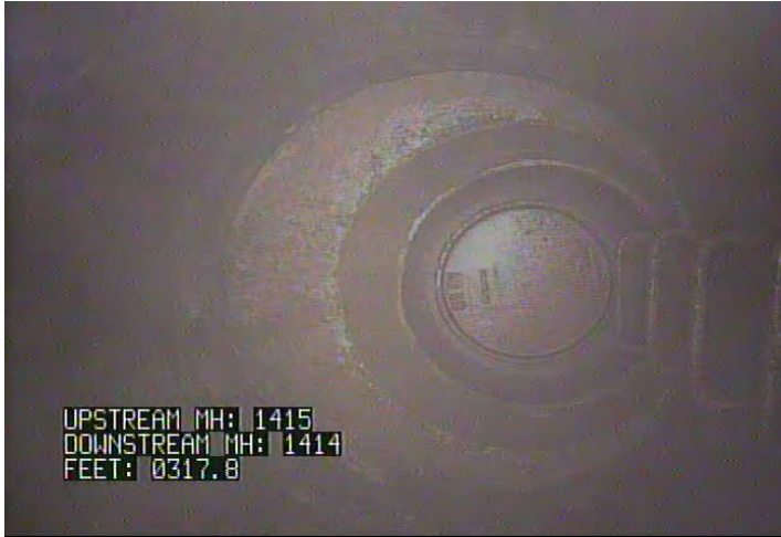
AMH - Access Point - Manhole @ 317.8 ft. MH 1414
