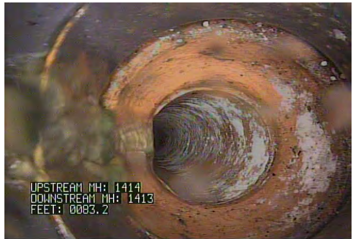
TFA - Tap, Factory Made: Active @ 83.2 ft. DYE PRESENT
