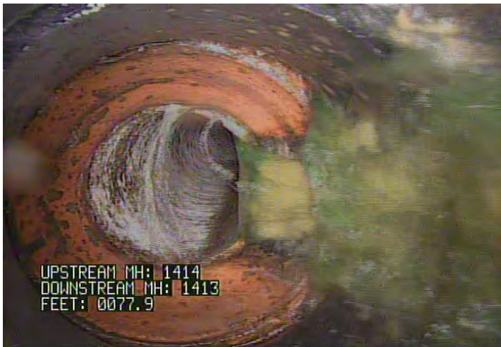
TFA - Tap, Factory Made: Active @ 77.9 ft. DYE PRESENT
