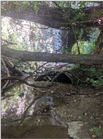
Figure 6. Outfall LC-145a, b
